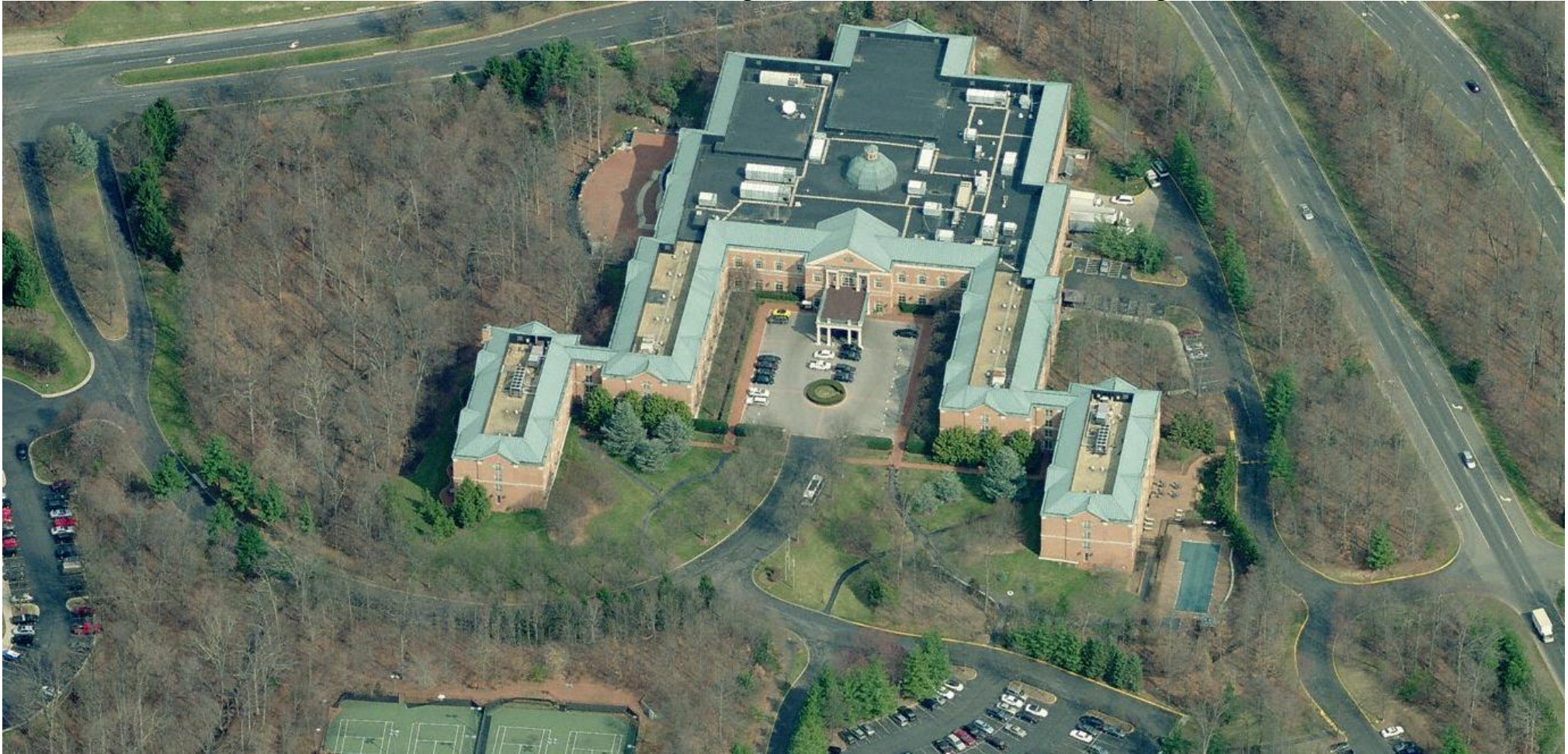
An aerial photo of the Westfields Marriott Hotel in Chantilly, Virginia, U.S.A., the site of the 2012 Bilderberg Meetings.
